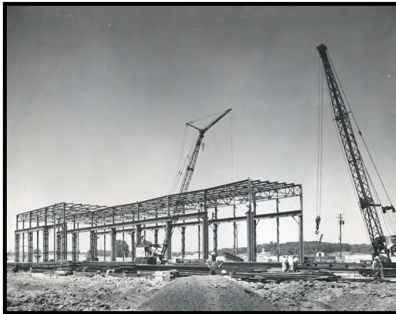
Figure 4: Steel Frame Erection for the X-700 Converter Shop and Chemical Cleaning Facility, May 1953
