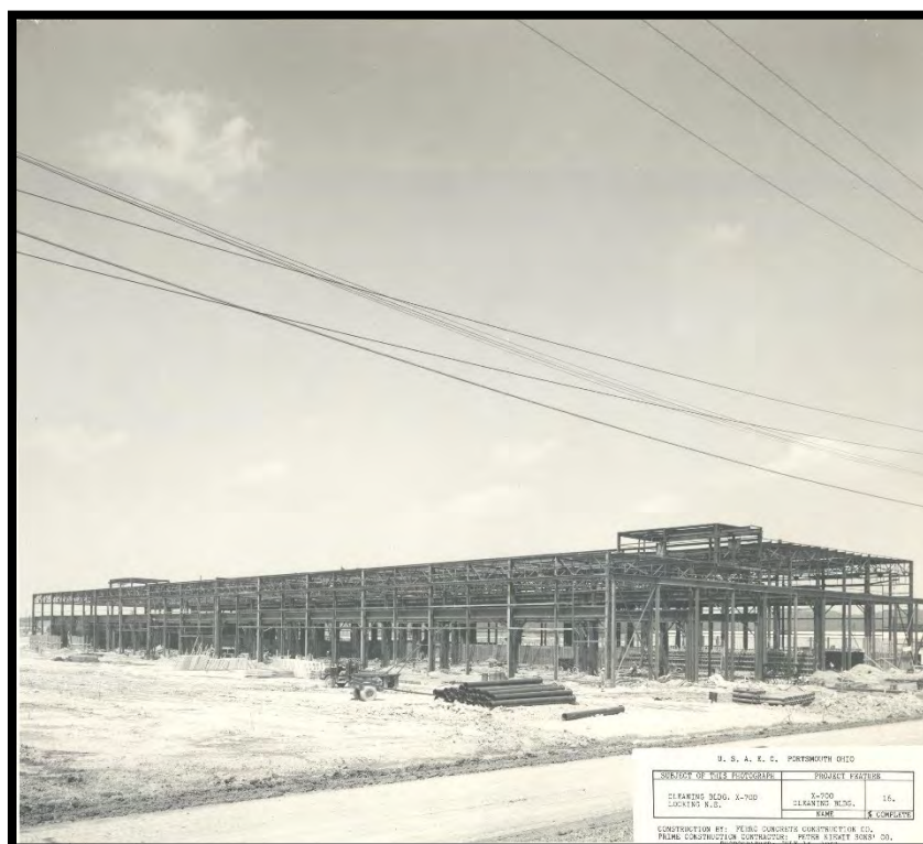
Figure 6: Steel Frame Erection for the X-700 Converter Shop and Chemical Cleaning Facility, Looking Northeast, July 1953
